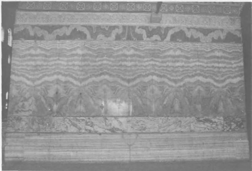
FIG. 13. — Views of the wall with crosses nos. 11-15 on plan at gallery level.
